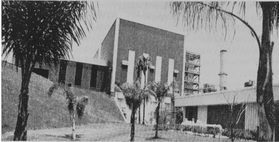
Figure 31 The Refuse to Energy Plant, a massive electricity-producing incinerator, burns 2,000 tons of garbage per day and generates $900,000 worth of electricity per month. Unfortunately, prevailing winds carry some of the mercury it releases into the atmosphere to the Everglades' ecosystem, which has become contaminated. Courtesy of the Pinellas County Commission.
