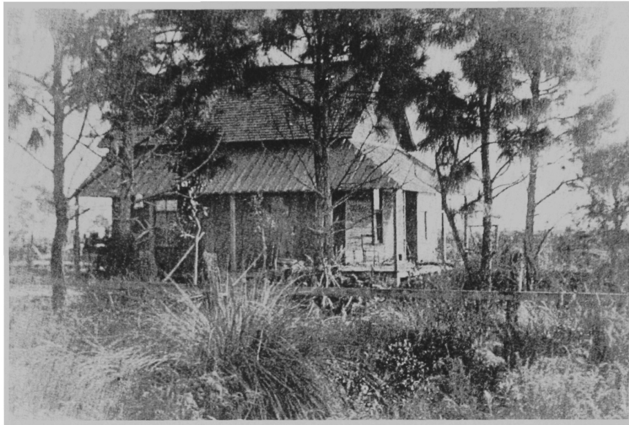
Figure 6 The traditional Cracker frontier home was designed to accommodate St. Petersburg's hot, humid climate. Courtesy of the St. Petersburg Historical Museum.
